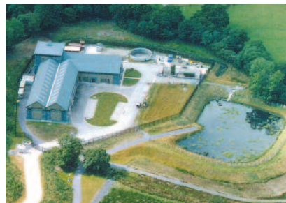
Example of remote pumping station.
